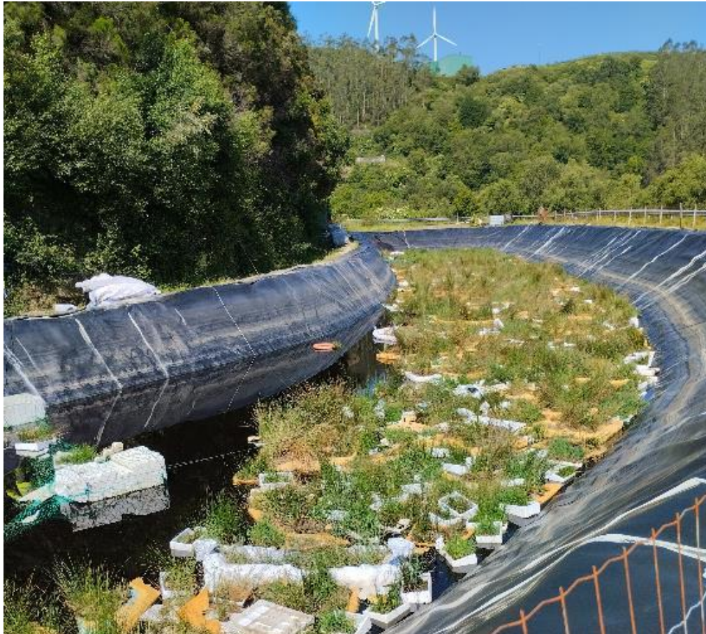
Figure 2. Floating treatment wetlands (FTW) at the LIFE GREEN ADAPT demonstration site in As Somozas, Spain (Source: LIMNOS Ltd).
