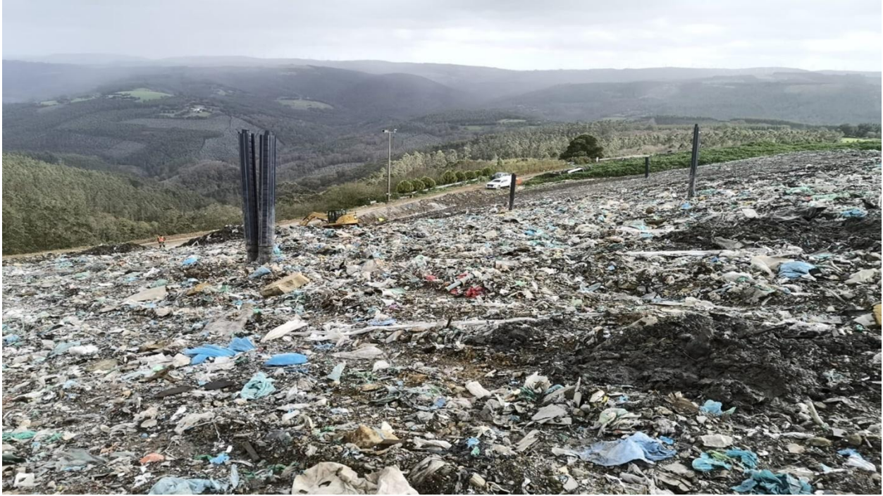
Xiloga landfill site at As Somozas, Galicia. Before the project. Photo Credit: Xiloga S.L.
